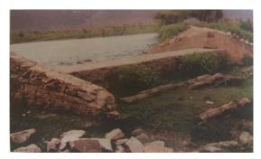
pit made by excavating the area and excavated soil is used to create wall on fourth side.
